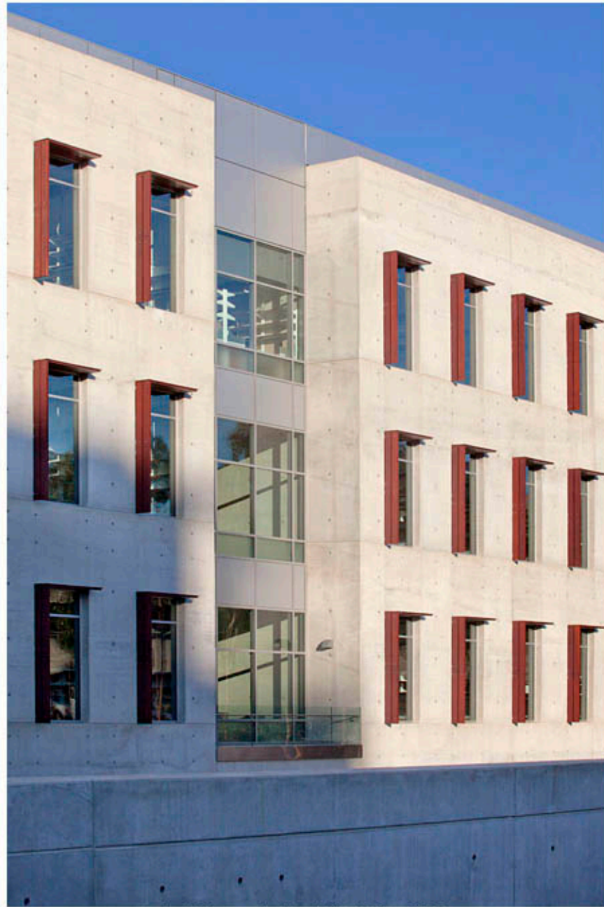
East Facade Detail 1947-JK.jpg
